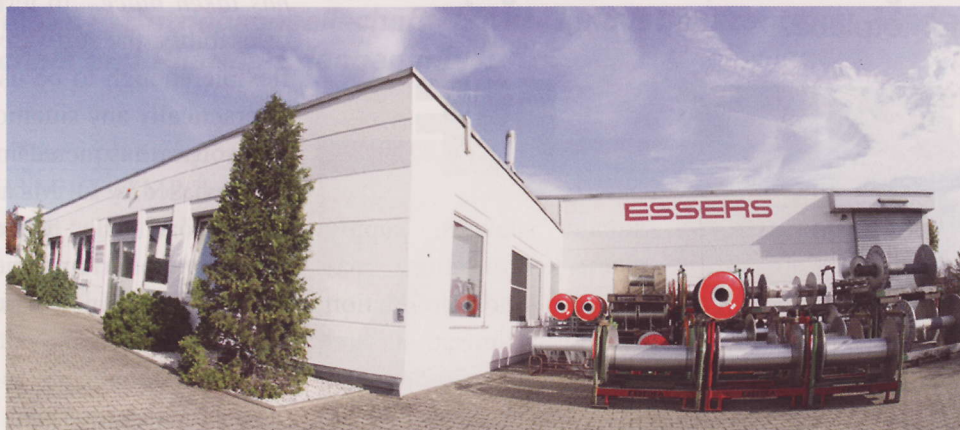
Heinrich Essers GmbH & Co. KG and Essedea GmbH & Co. KG operate state-of-the-art production facilities in the German town of Wassenberg
